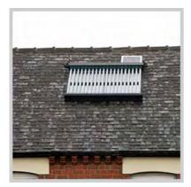
Figure 9 - Solar water heating panels.
