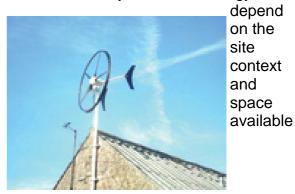
Figure 12 - Micro wind turbine attached to residential dwelling
