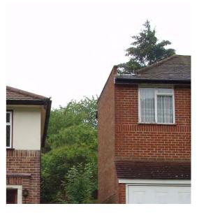
Fig 30 - An example of a parapet built to avoid an eaves and gutter overhang. This should be avoided.
