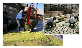
Figure 17 - The laying of an extensive green roof. Sedum Blankets rolled on top of a felt roof.
